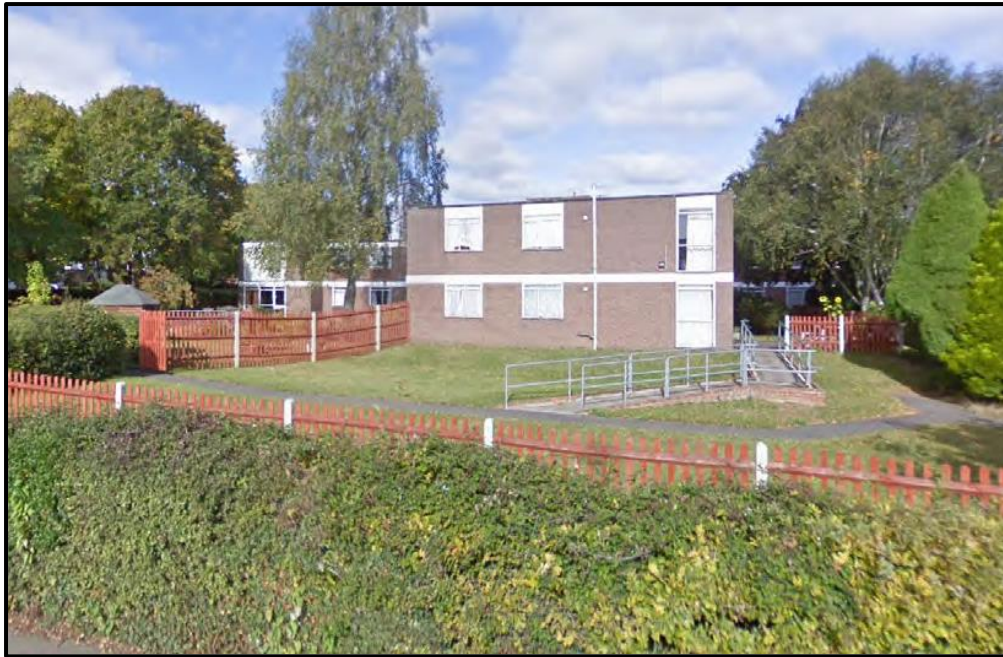
Fig A-2.2: Brockhurst Care Home – Previous Development. Slade Road Elevation 20+ metres from boundary..
