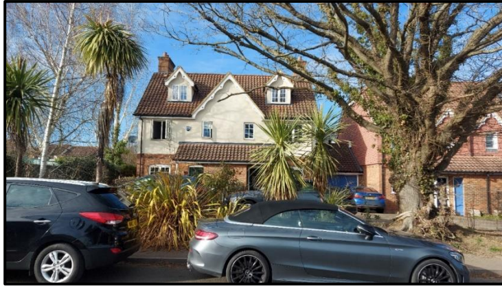
Fig A-1.7: Slade Court adjacent Brockhurst Site
