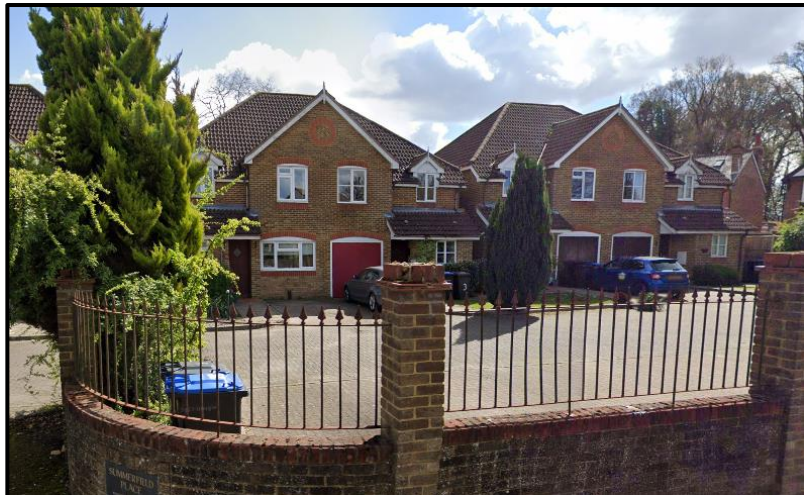
Fig A-1.4: Crawshaw Road Properties adjacent to site.
