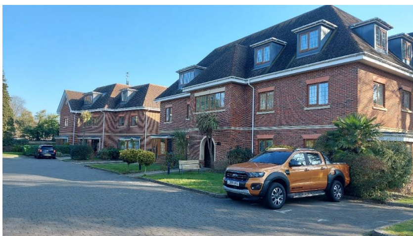
Fig A-4.1: Feature Brickwork, stone lintels, attractive fenestration, pitched roof with part dormers.
