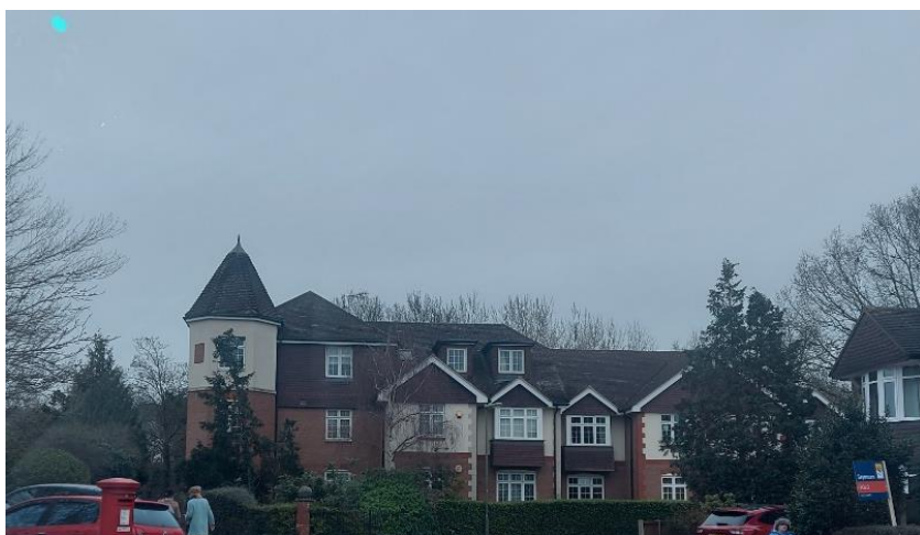
Fig A-4.2: Tower feature, Feature Brickwork, tile hanging, pitched roof.
