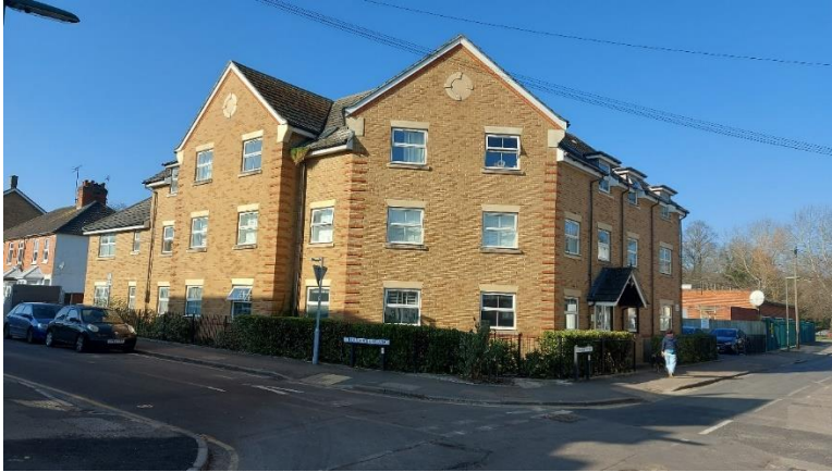
Fig A-4.3: Feature Brickwork, stone lintels, attractive fenestration, pitched roof with part dormers.
