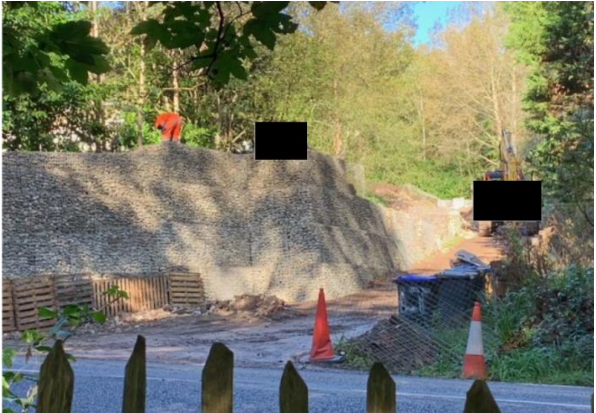
Fig 3: Site frontage (part) onto Chobham Road after introduction of walls & piling.
