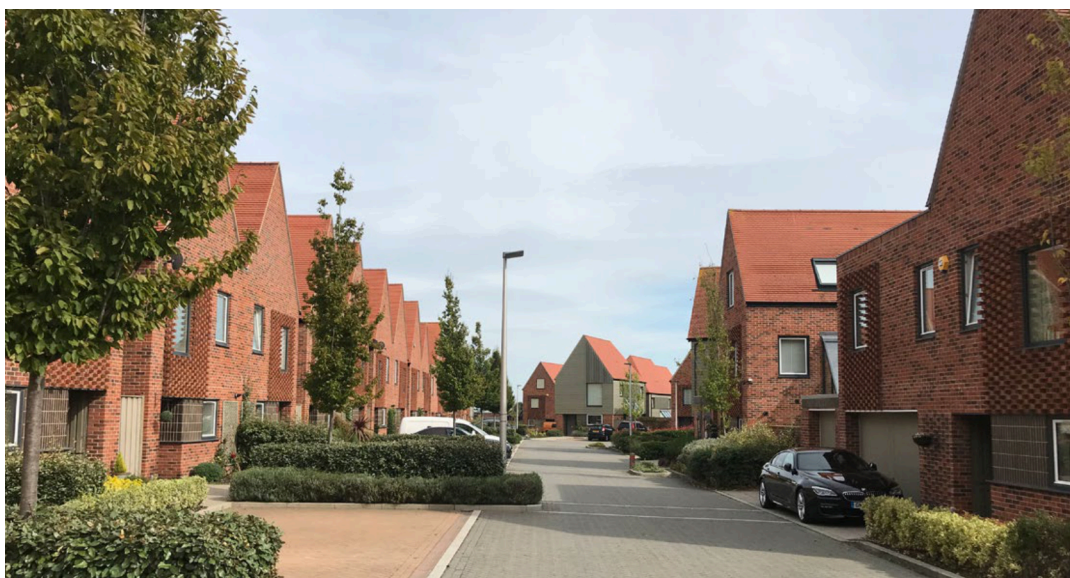
Fig 6.13 - This street is designed with parking bays broken up and screened with robust shrub planting and small trees (NDG p.25)
