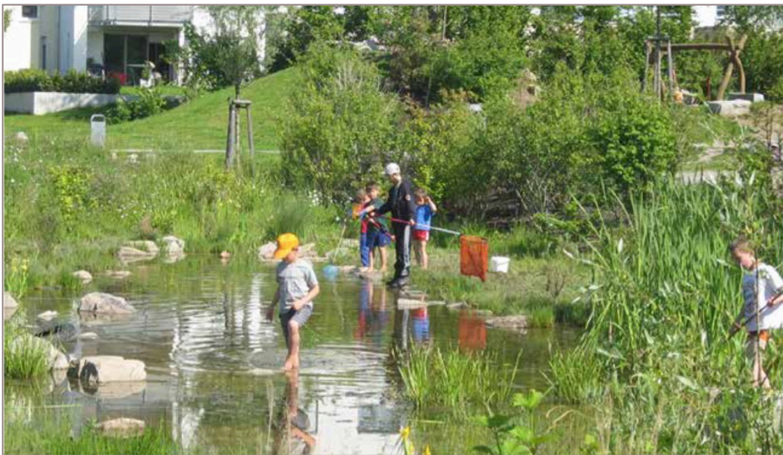
Fig 6.17 - Shallow slopes, low water depth and stable edges minimise the need for fences and illustrate a design led approach to health and safety.
