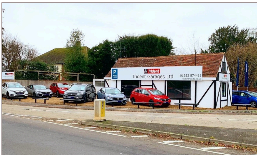
Fig. 9.8 – Old Forge Building, Guildford Road.
