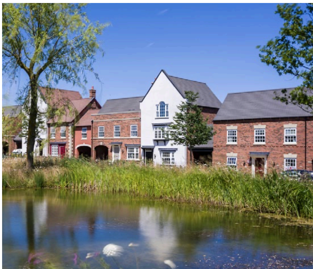
Fig. 6.1 – Example of a new development which integrates sustainable drainage and biodiversity habitat. (NDG)
