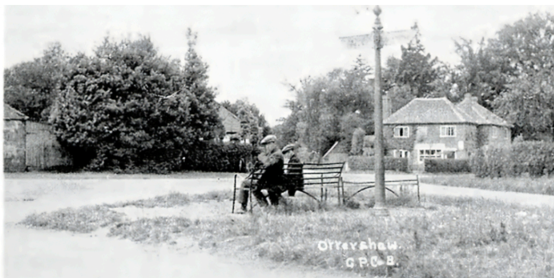
Fig 2.1 – Ottershaw 1919 at the location of the A320 Otter Roundabout.
