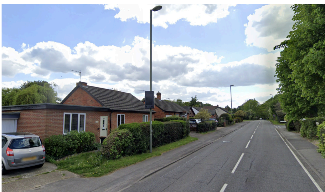
Fig 5.6 – Chobham Road Street scene
