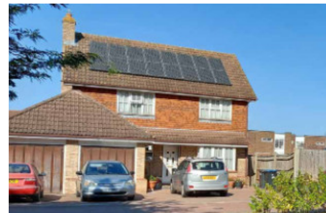
Fig.62 Property built with gable roof with retrofitted photovoltaic on roof
