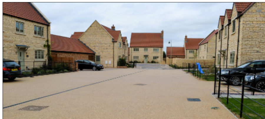
Fig.82 An example of resin bound surfacing (Source:www.sureset.co.uk)
