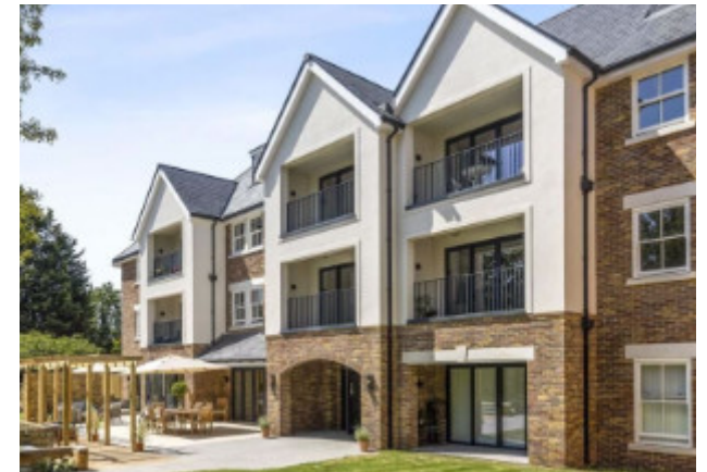
Fig.64 Apartment block using high quality materials and massing broken down with projections and recesses to avoid monolithic bulk
