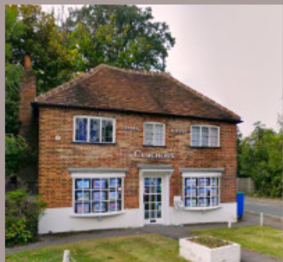
No.2, Chobham Road, Grade II, building
