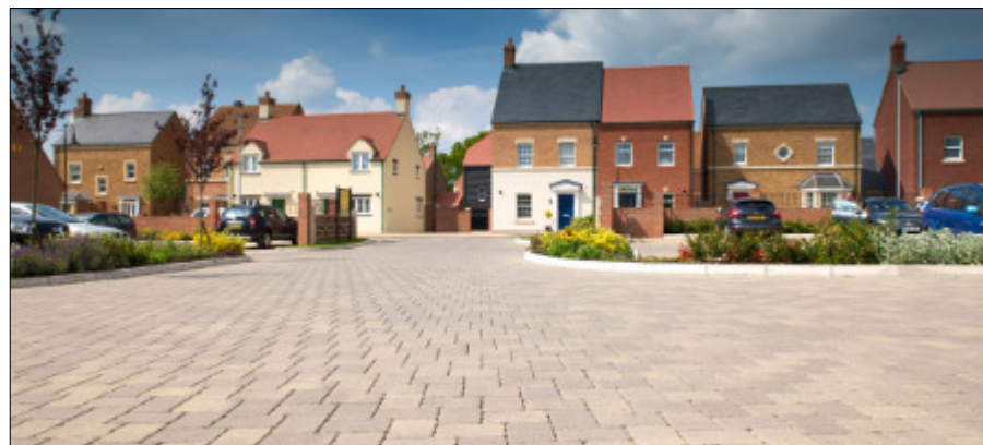
Fig.81 An example of permeable pavers (source:www.marshalls.co.uk)
