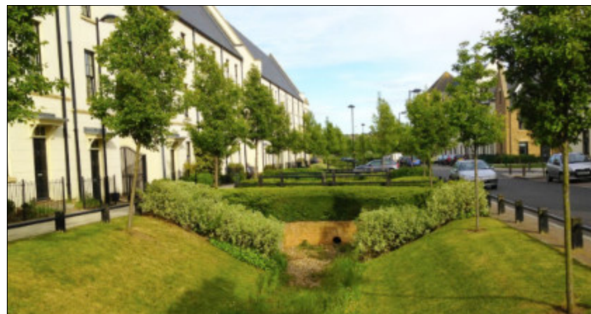
Fig.79 Example of swale integrated within a development contributing to Green and Blue infrastructure on the site.
