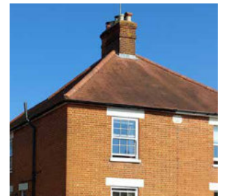
Hipped roof with clay tile
