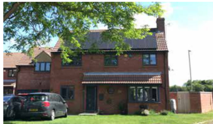
Fig.74 Solar panels on existing home
