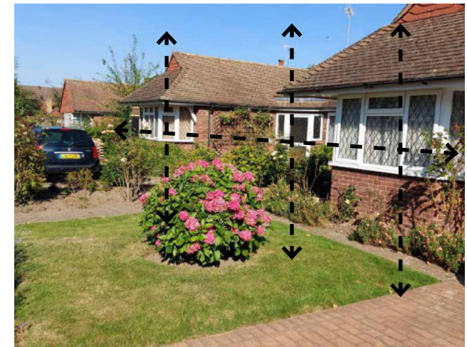
Fig.61 Windows spaced evenly along the building elevations in a low density area in the village
